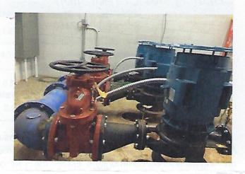
Booster Station Improvements water pumping capacity increased by 20 %, with Energy reductions of 25 %. Rocky Hill booster below . improves water pressure and water quality to Spencer residences.
