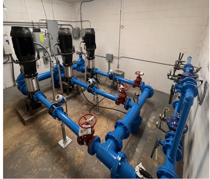
West Booster Pump Station, new high efficiency pumps and new electrical VFD's installed in 2023
